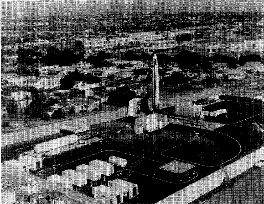
Douglas Aircraft built a mockup Thor launch facility at its Santa Monica plant in 1958. With the exception of the truncated missile shelter, the support equipment shown in the photograph was all standard equipment.
