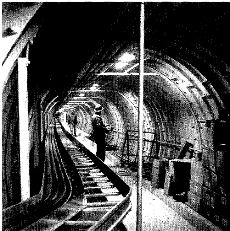
In this 1960 photograph, work on the main tunnel of the Titan I launch complex at Vandenberg AFB nears completion. Forty feet beneath the surface, the tunnel connected the control center to the missile silos.
