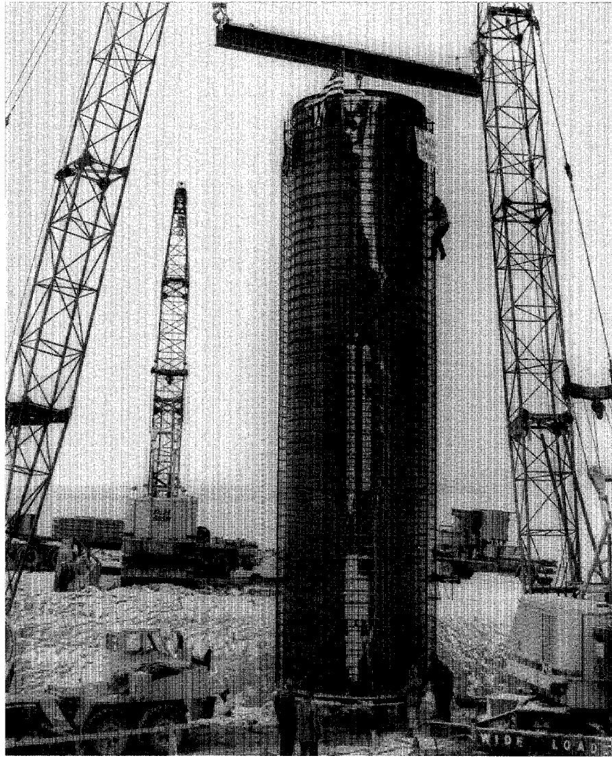
Workers from U. S. Steel's American Bridge Division put the finishing touches on the last of more than 100 silo liners it installed in Minuteman launch facilities around Malmstrom AFB, Montana.
