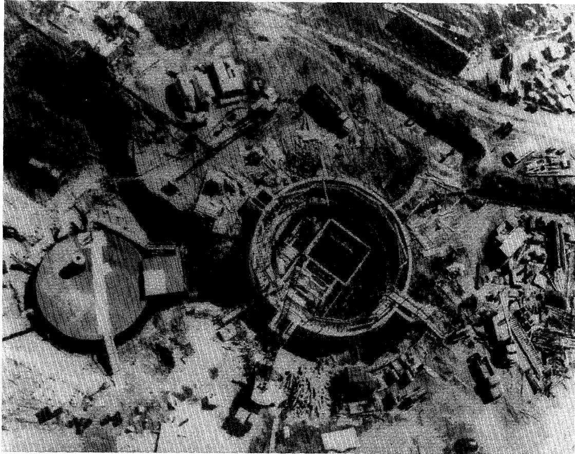
An overhead view of an Atlas F silo under construction near Plattsburgh, New York. The launch control center is on the left. The steel crib that supported the missile and its ancillary equipment is nearing completion.
