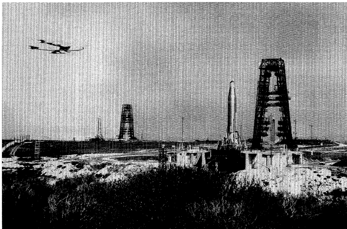
This 1960 photograph shows two Atlas D ICBMs deployed on open launch pads at Vandenberg AFB, California. This was a stopgap measure, intended to serve only until the protected, horizontal launchers were ready.
