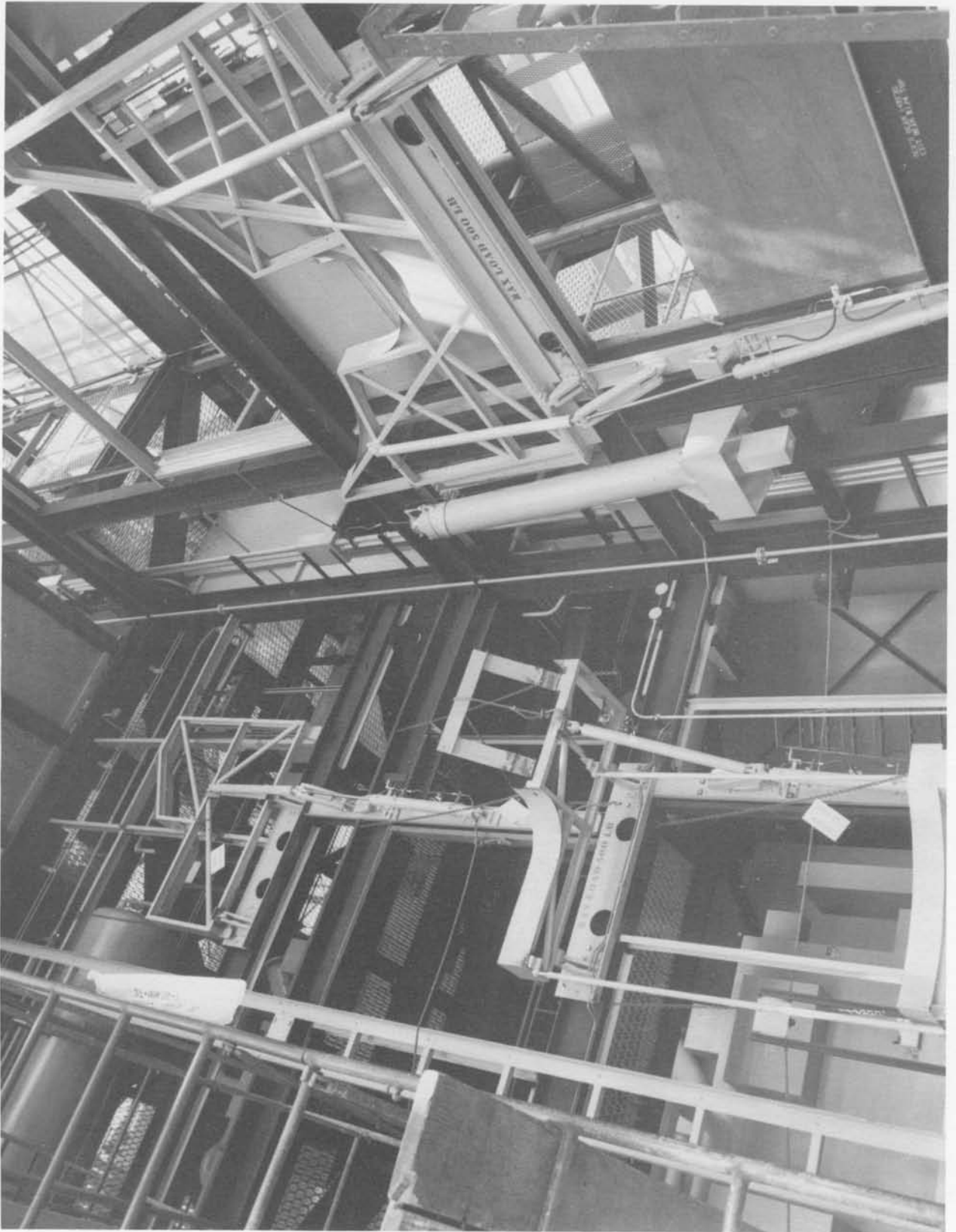
Collimator and work platforms (Neg. No. 53915A dated 8-16-60).
