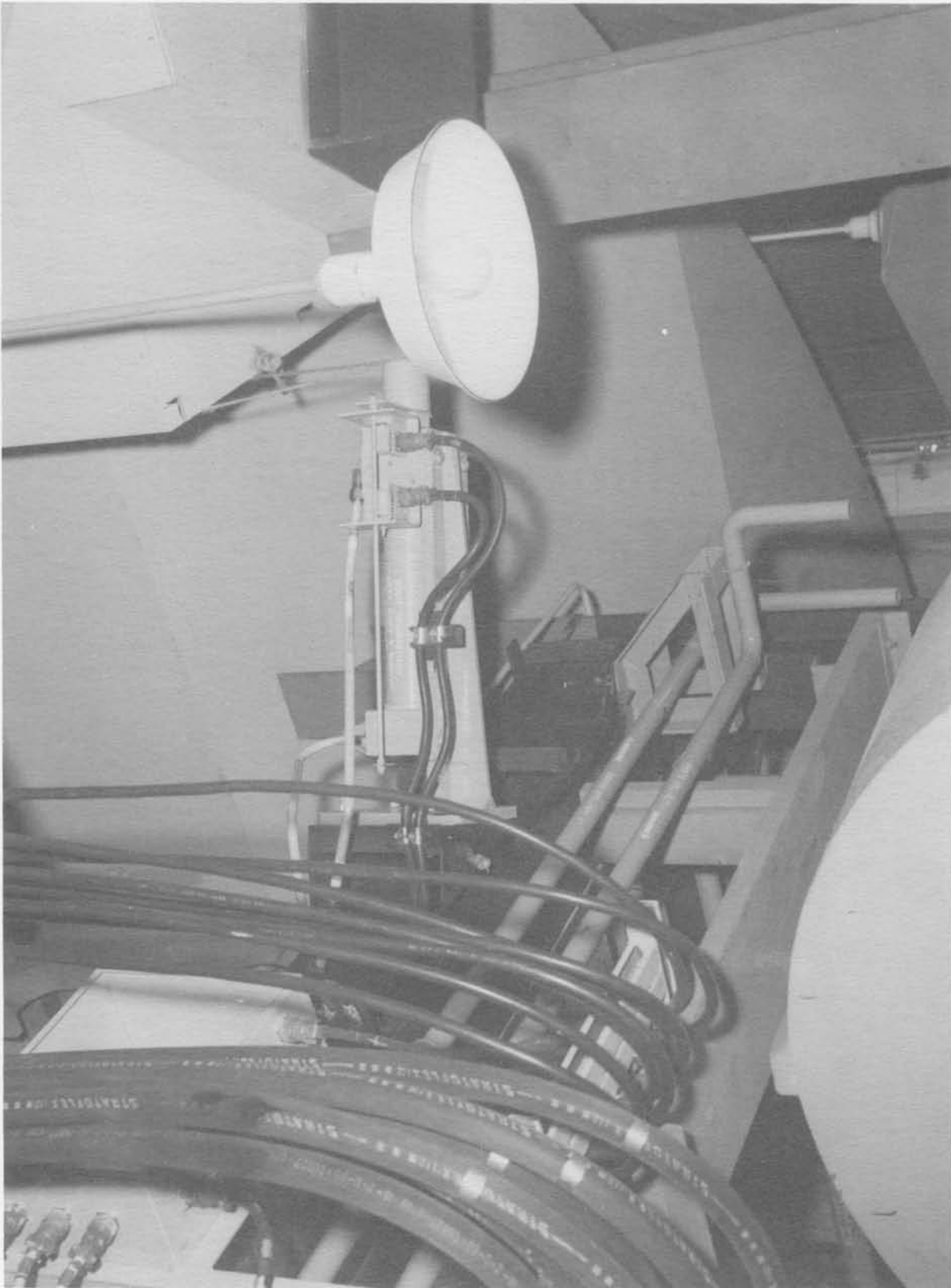
Horizontal crib lock at Column A (Neg. No. 66253A dated 3-23-61).
