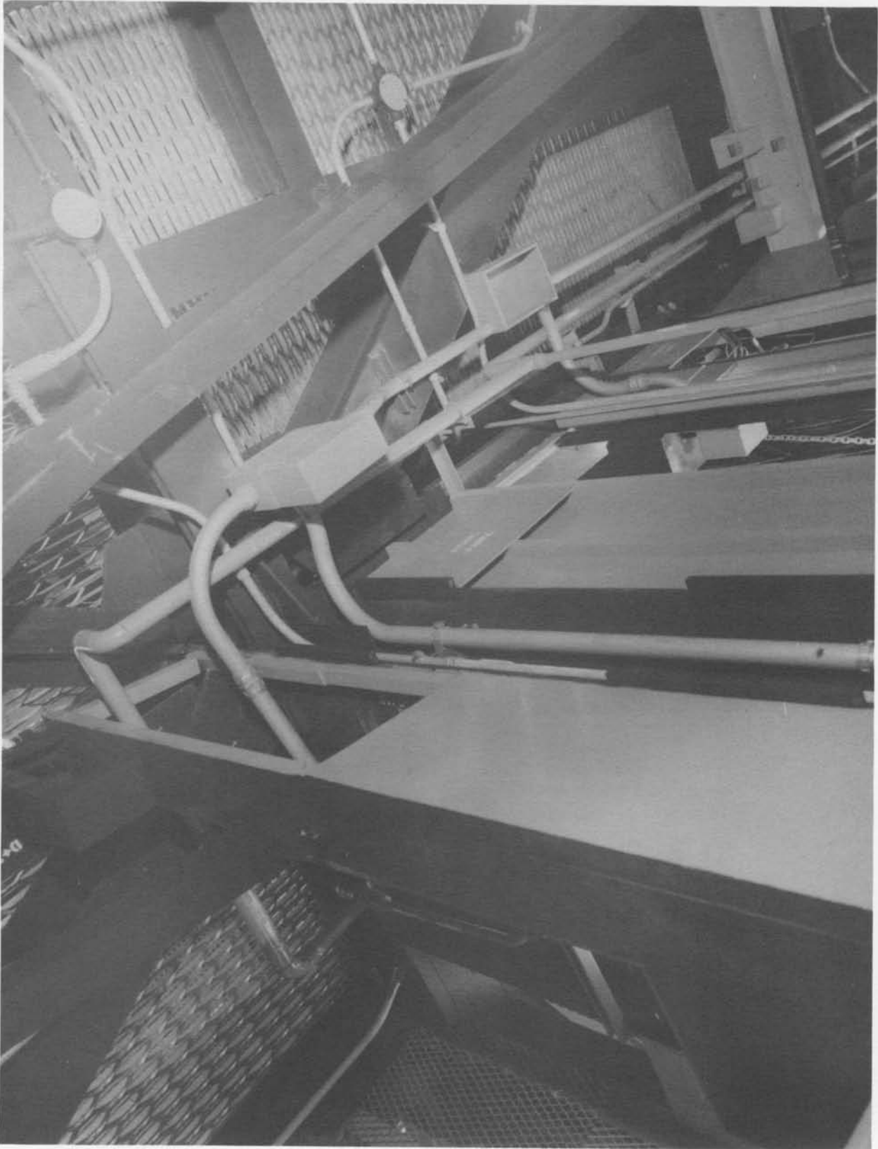
Looking up from Column J (Neg. No. 68073A dated 4-27-61).
