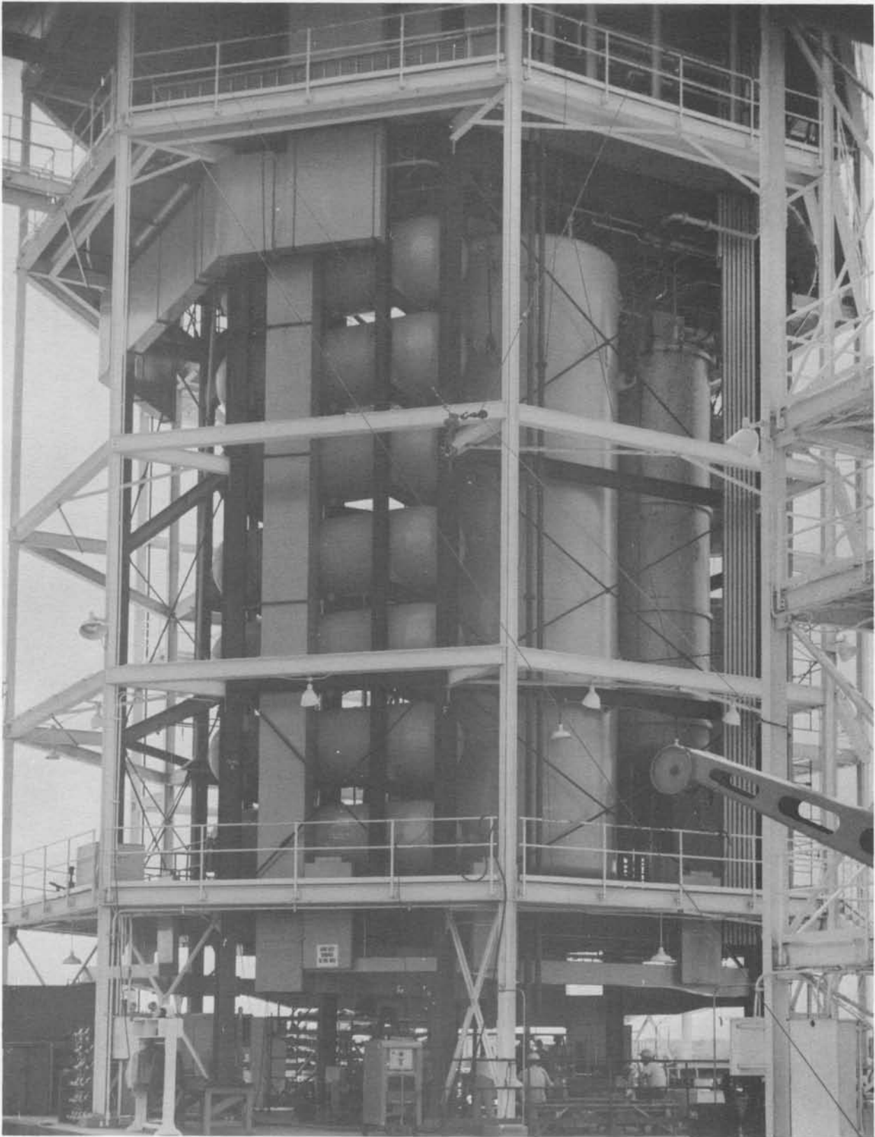
Tank farm from ground (Neg. No. 53923A dated 8-16-60).
