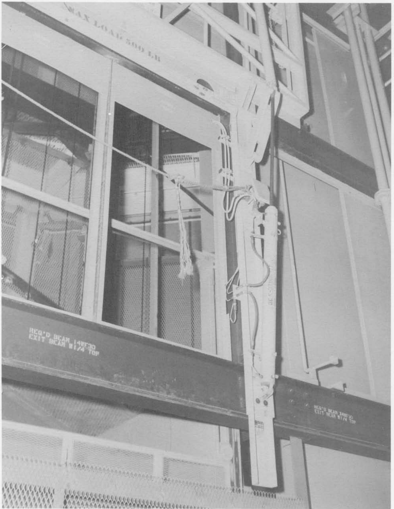
Work platform tubes, north (Neg. No. 66231A dated 3-23-61).
