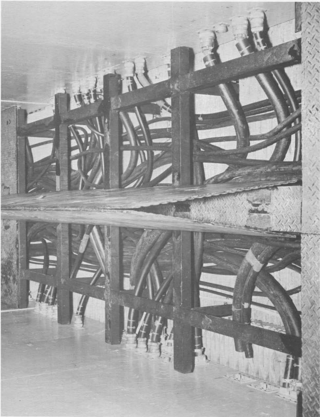
Cables under steel deck logic No. 2 to responder No. 2 (Neg. No. 55771A dated 9-27-60).
