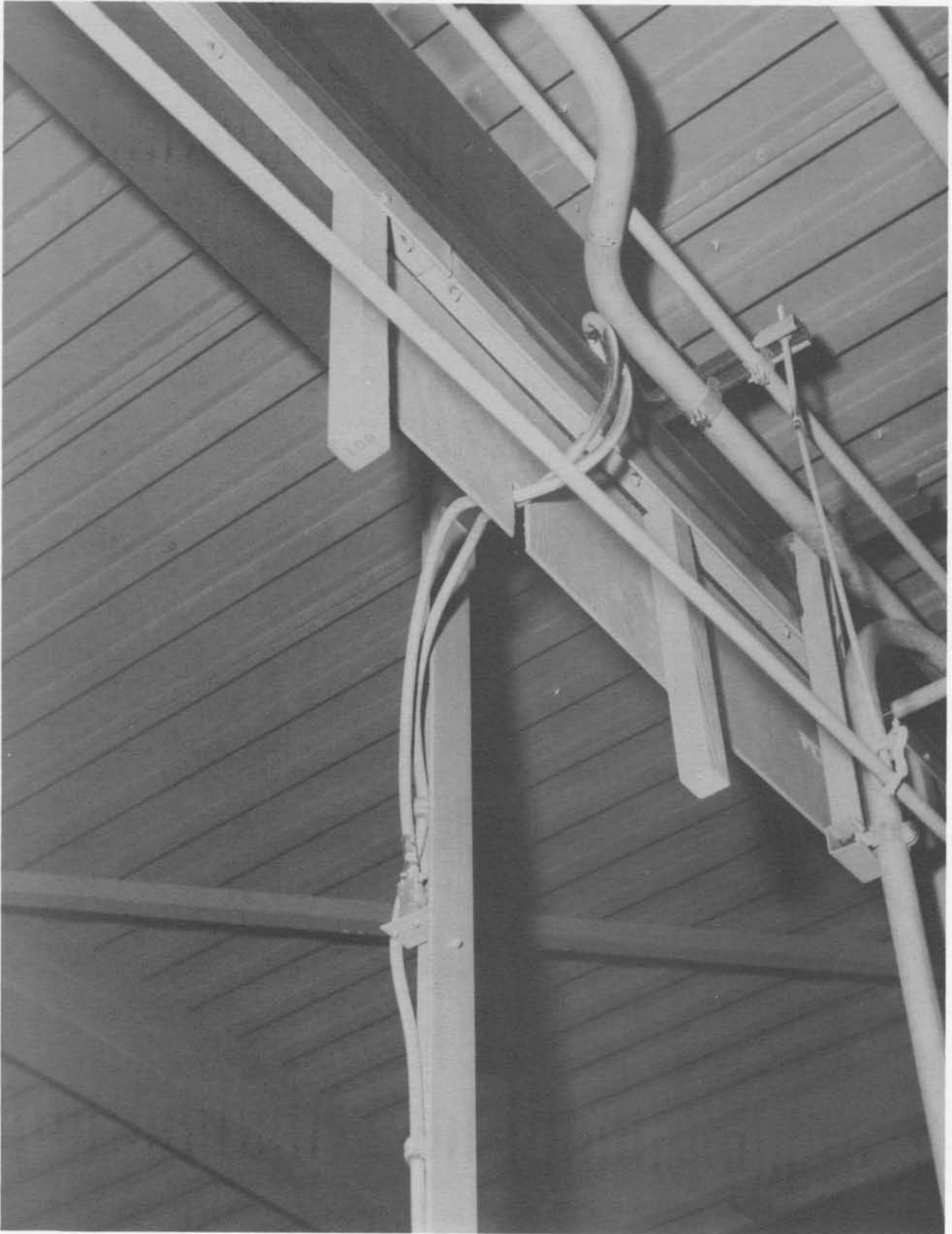
Guide rail cables, west side (Neg. No. 67361A dated 4-14-61).
