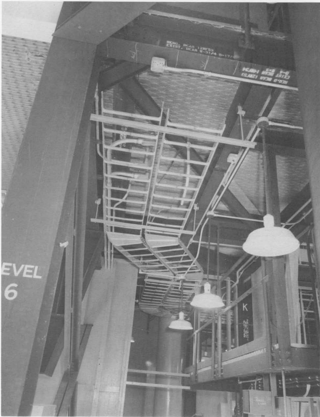
Looking up and west from near Column D (Neg. No. 68077A dated 4-27-61).
