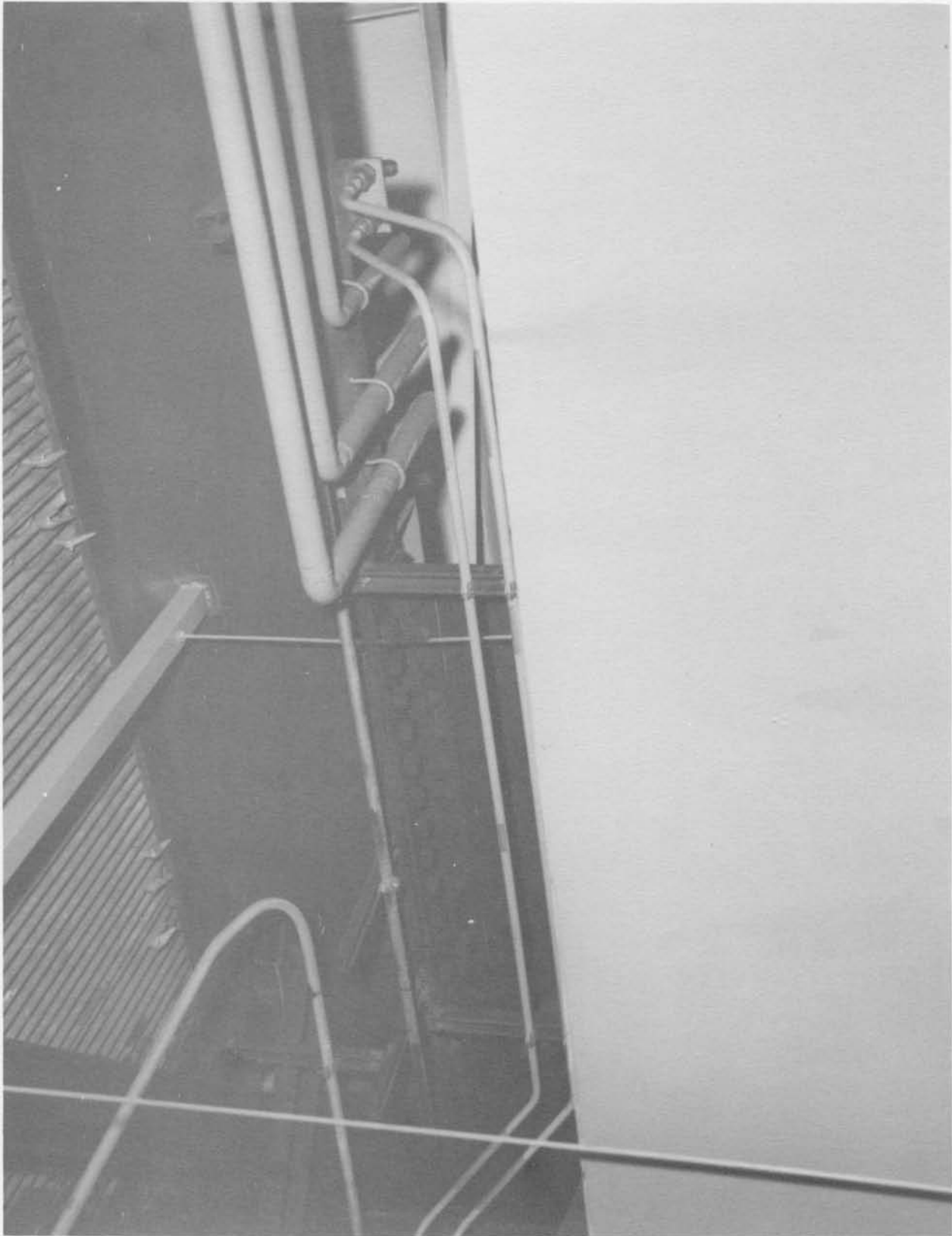
Hydraulic tubes at south side (Neg. No. 64934A dated 2-27-61).
