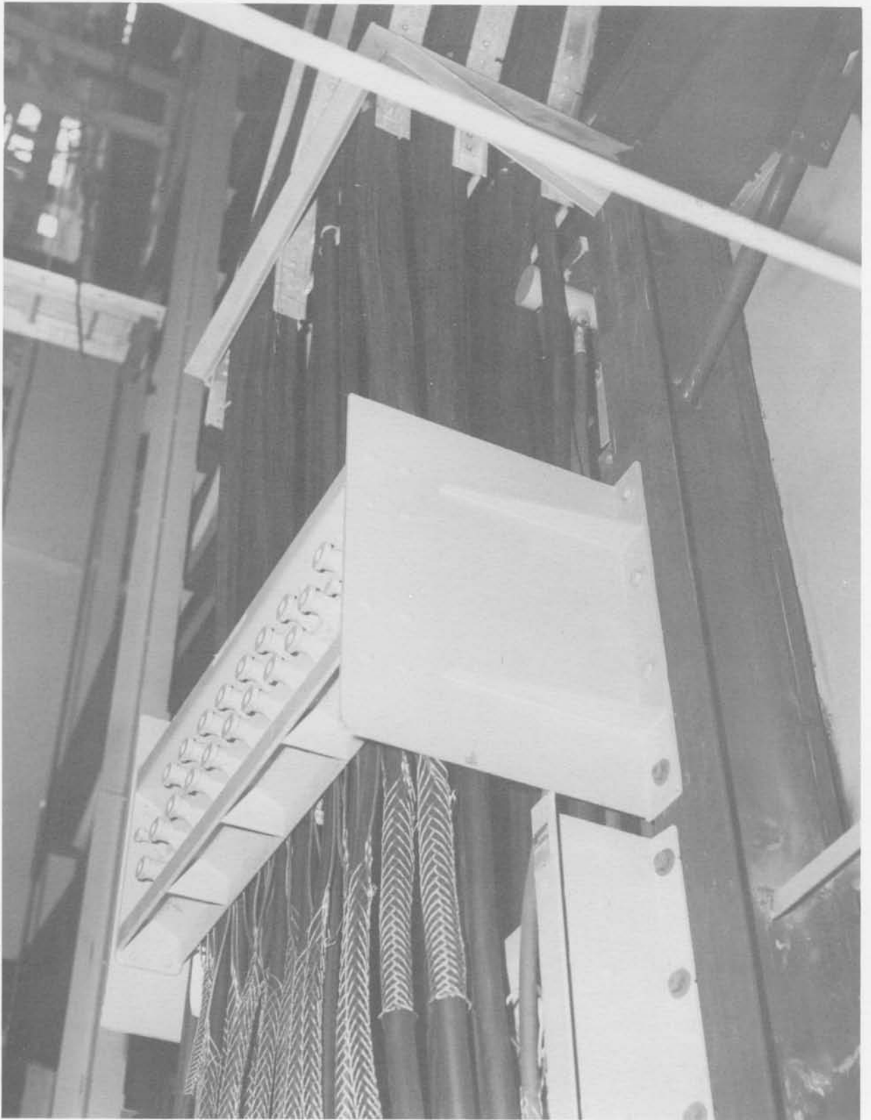
Cable loop bracket (Neg. No. 67330A dated 4-14-61).
