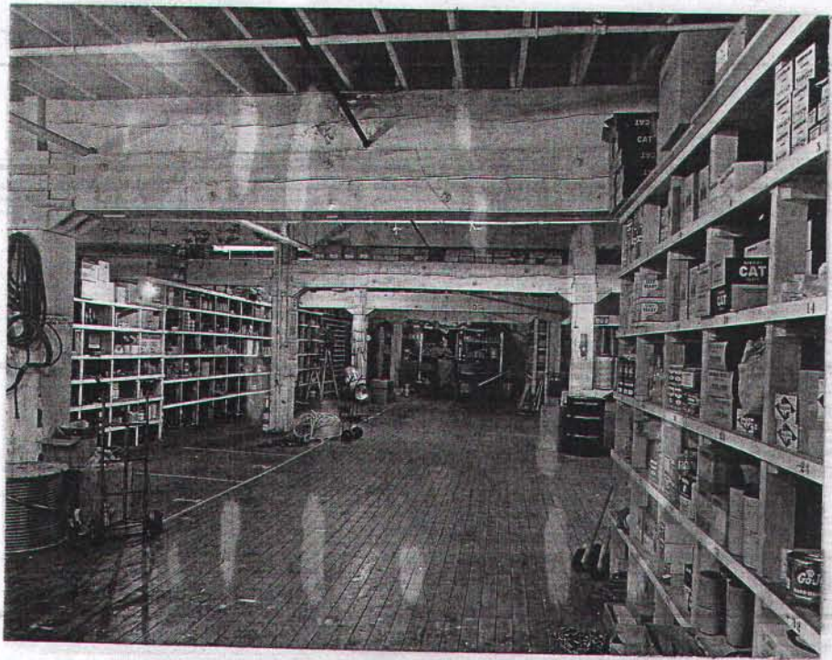
View of one of Western Contracting Corporation's buildings used during construction. It also served as their warehouse.
