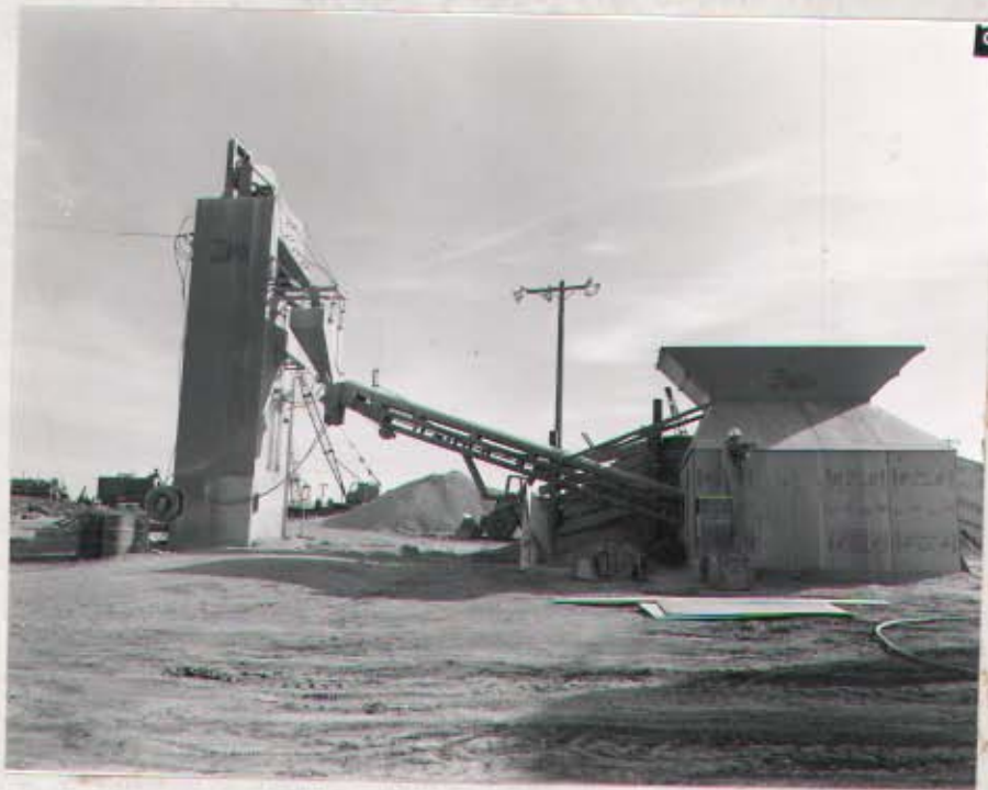
SITE 9, BRAINARD, NEBRASKA. 3 Aug. 60. #39152. Two views of Contractors Batch Mixing plant at Site. SITE 9, BRAINARD, NEBRASKA. 3 Nov. 60. #41862
