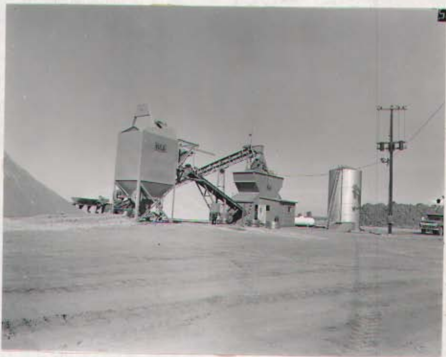
SITE 7. YORK, NEBRASKA. Contractors batch mixing plant. #41857.
