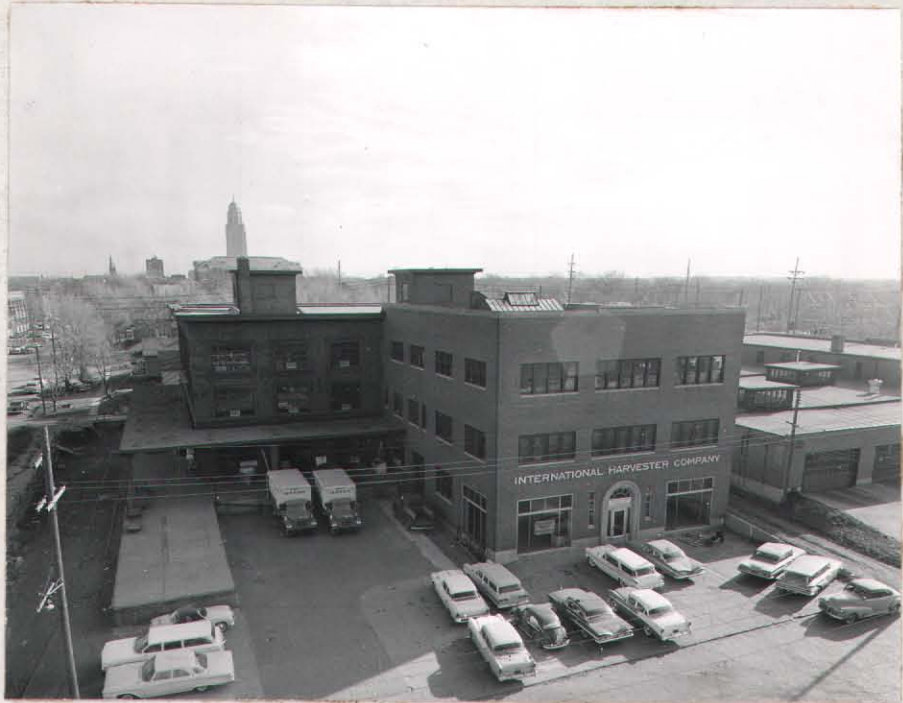
View of Western Contracting Corporation Building utilized by their engineering department.
