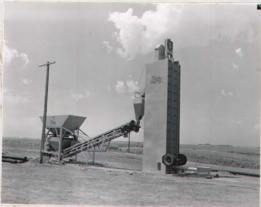
SITE 9, BRAINARD, NEBRASKA. 3 Aug. 60. #39152. Two views of Contractors Batch Mixing plant at Site. SITE 9, BRAINARD, NEBRASKA. 3 Nov. 60. #41862
