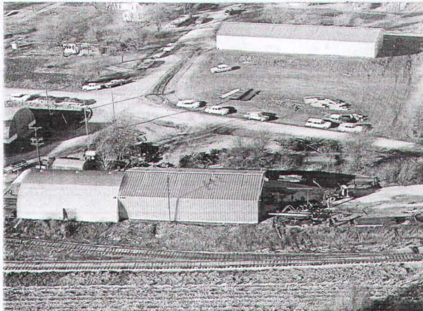
902. Aerial view to the northeast shows the Cortland, Nebraska pipe shop and storage area. Contractor leased the right half of the long center structure for this work and storage area is shown to the right of building. Note long joint of large diameter pipe being handled by winch truck.
