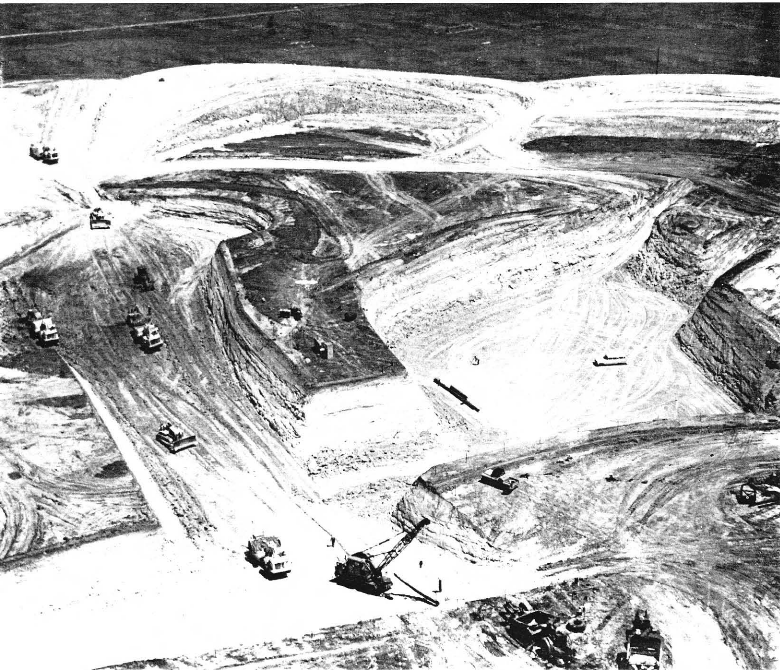
Excavation of the first Titan site at Lowry AFB, CO.
