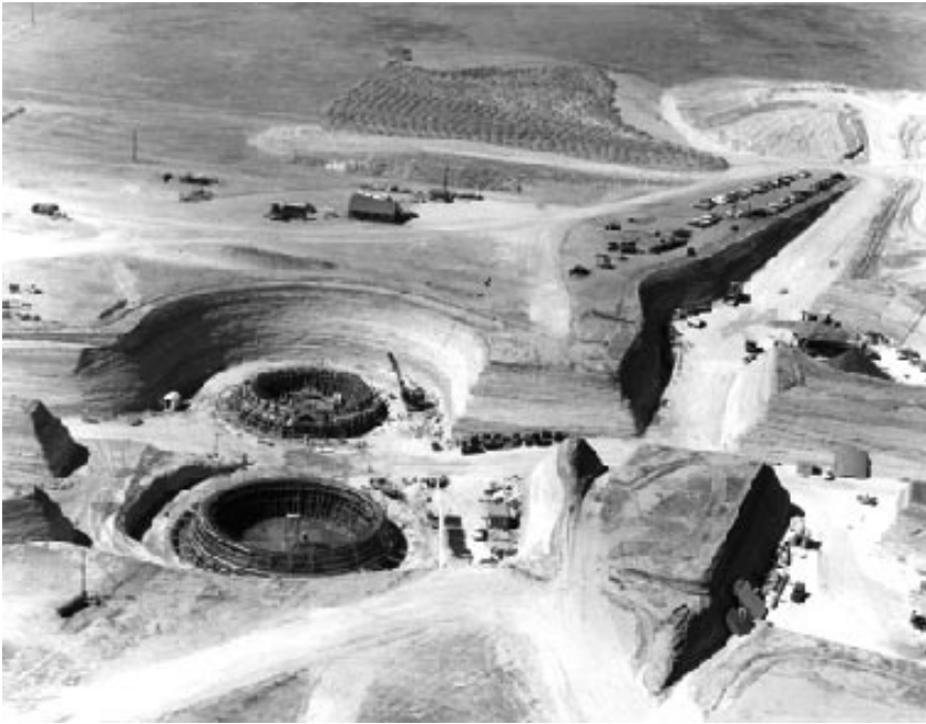
A missile silo construction site.
