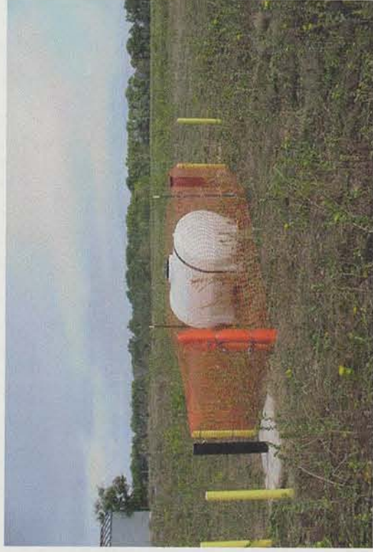
MW08 & MW09 – Poly tank for temporary storage of development water.
