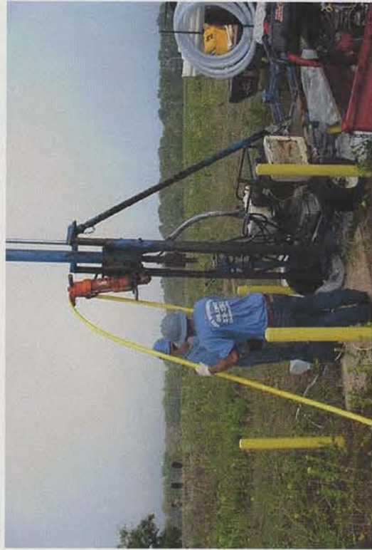
Pulling \frac{3}{4} horse electric pump from MW09.
