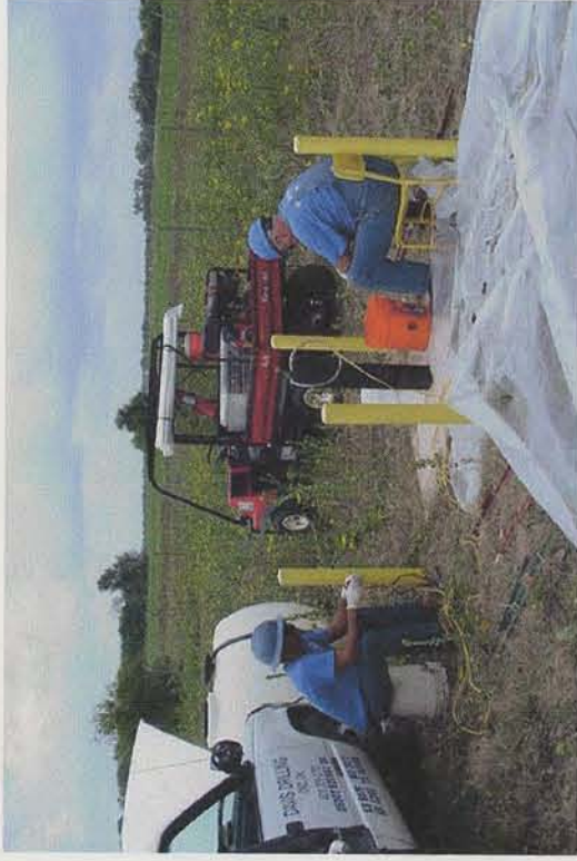
MW08 Redevelopment – Electric pump run from truck battery.
